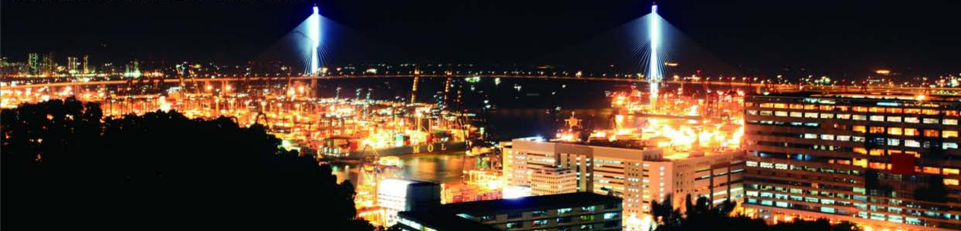
STONECUTTERS BRIDGE - HONG KONG
